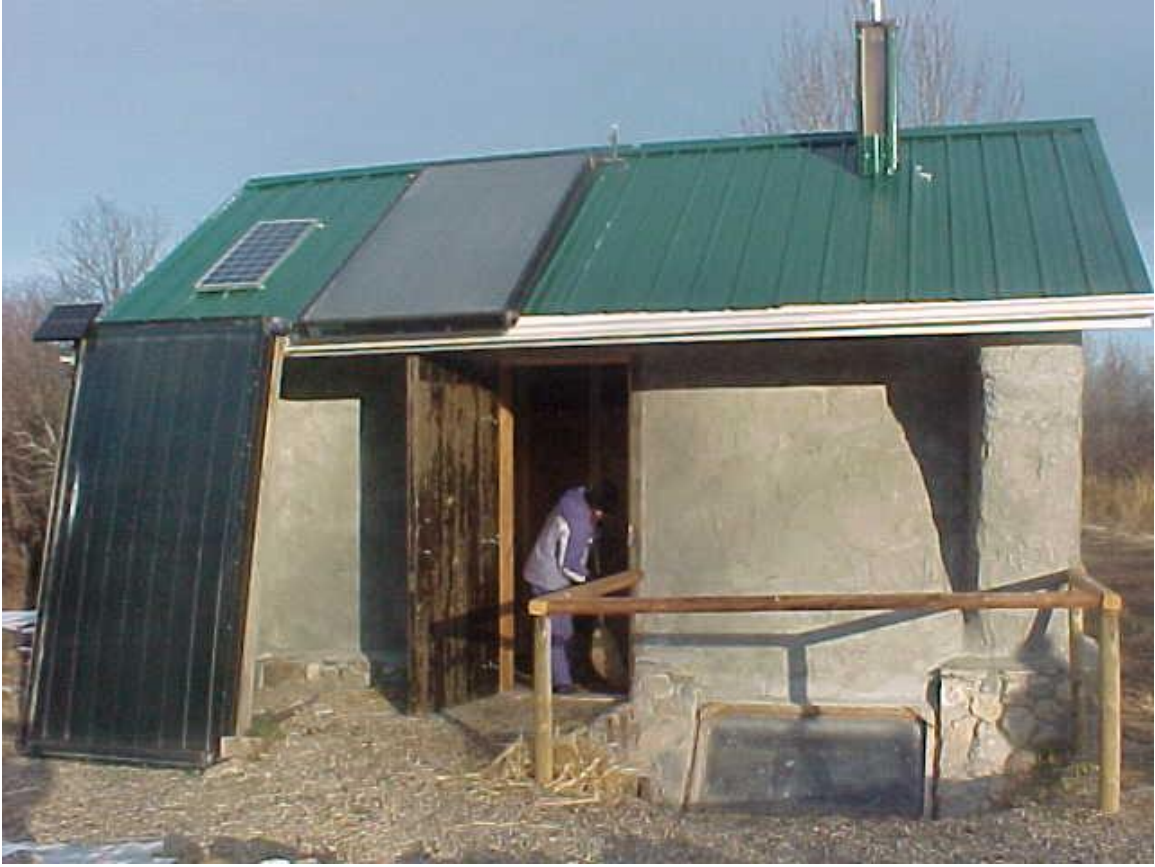
The toilet is ready to use.
